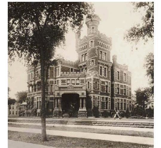
Fig. 5. The Palmers' home, "The Castle," at 1350 North Lake Shore Drive, 1890/1910. Institutional Archives, Art Institute of Chicago.
